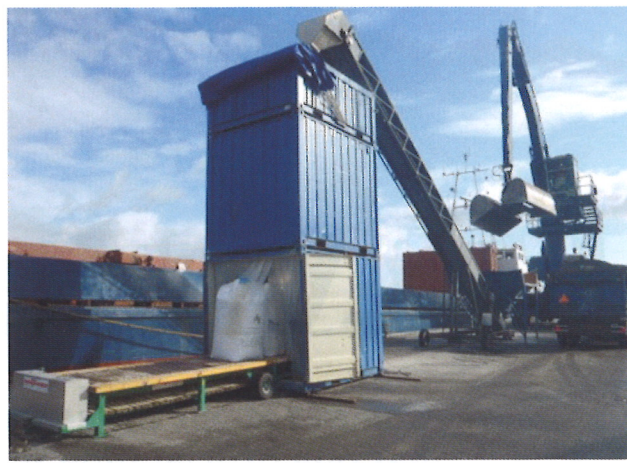
Figure 4. Portable triple container set-up at the side of a ship to transfer bulk fertilizers out of the ship into big bags at the key side.
